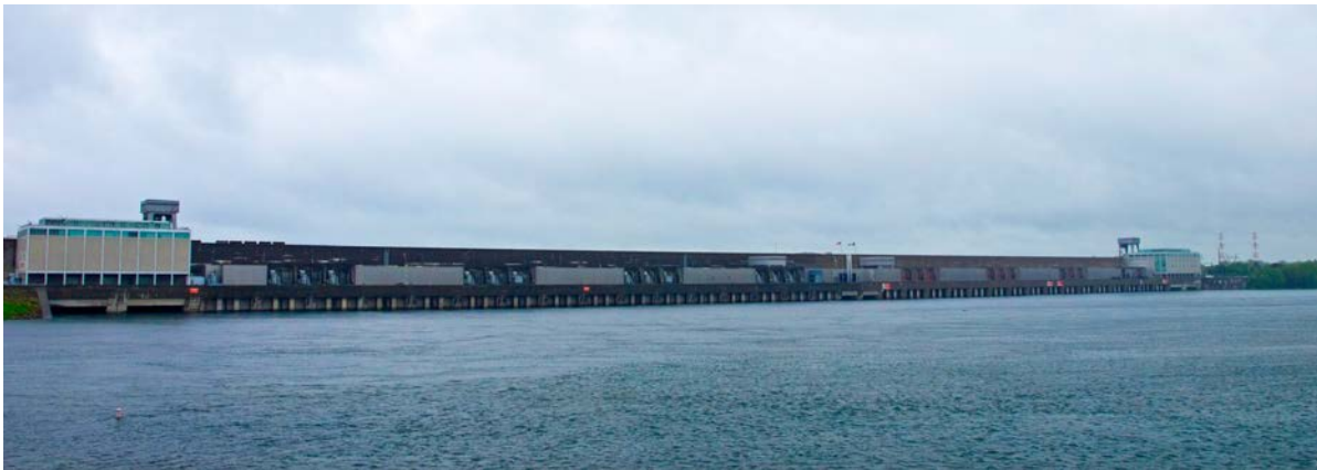
ORMEUS COIN EXPANDS WITH COST-EFFECTIVE POWER FROM HYDRO DAM ON AMERICAN/CANADIAN BORDER
